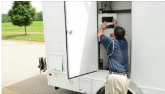
Removing Fuse Panel
