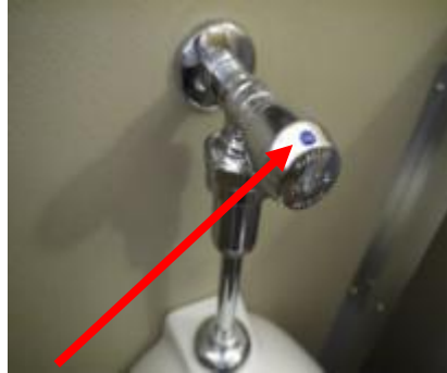
2. Remove Cap and Screw with Allen Wrench.
