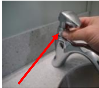
2. Remove Fastener
