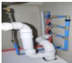
Location of Urinal Shut Off Valve in Service Area.
