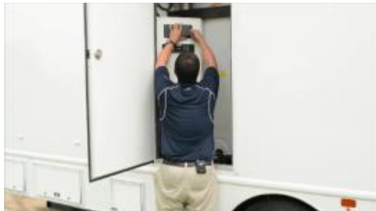
Removing Fuse Panel
