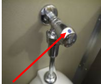
2. Remove Cap and Screw
