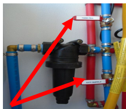
Tank Fill Valve Open and City Valve Closed
