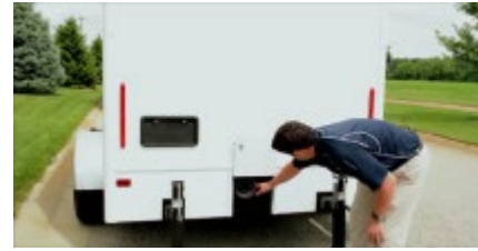
Accessible 4" Clean Out Port.
